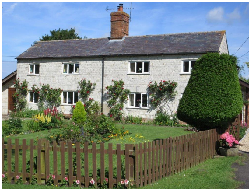
Figure 18 – Typical Slate Roofed Cottages
