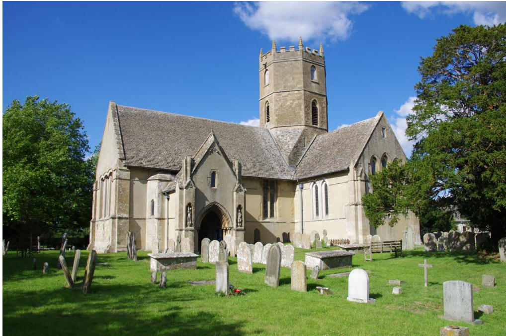
Figure 12 – St Mary's Church Uffington
