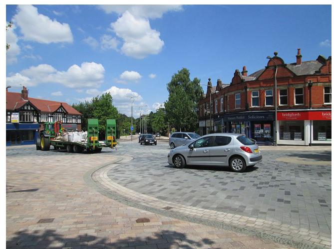
Example of dropped curb, making the pedestrian priority area inclusive for all users
