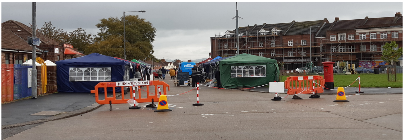
Temporary street closure of Barnstaple Road,
