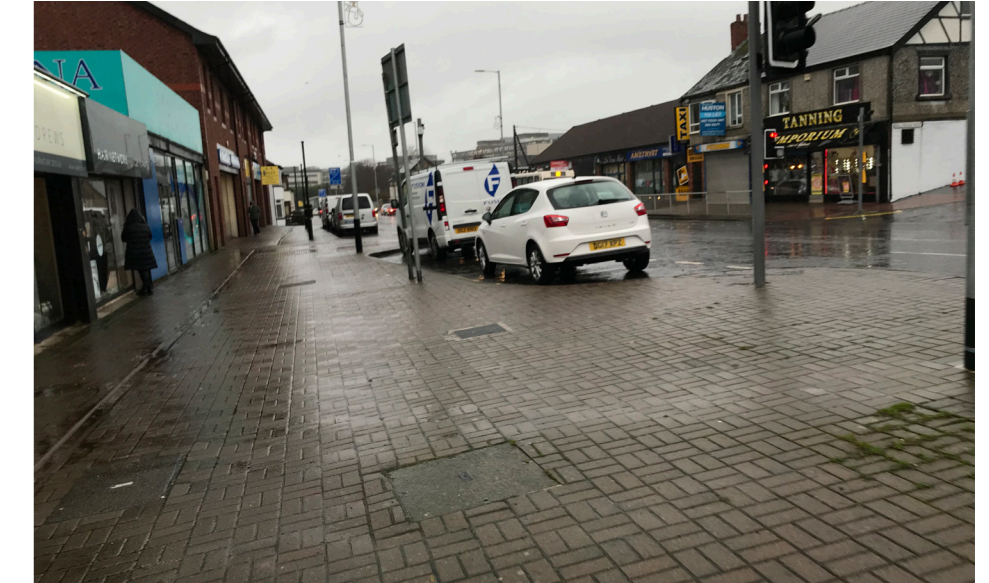
View of existing paving along Upper Newtownards Road
