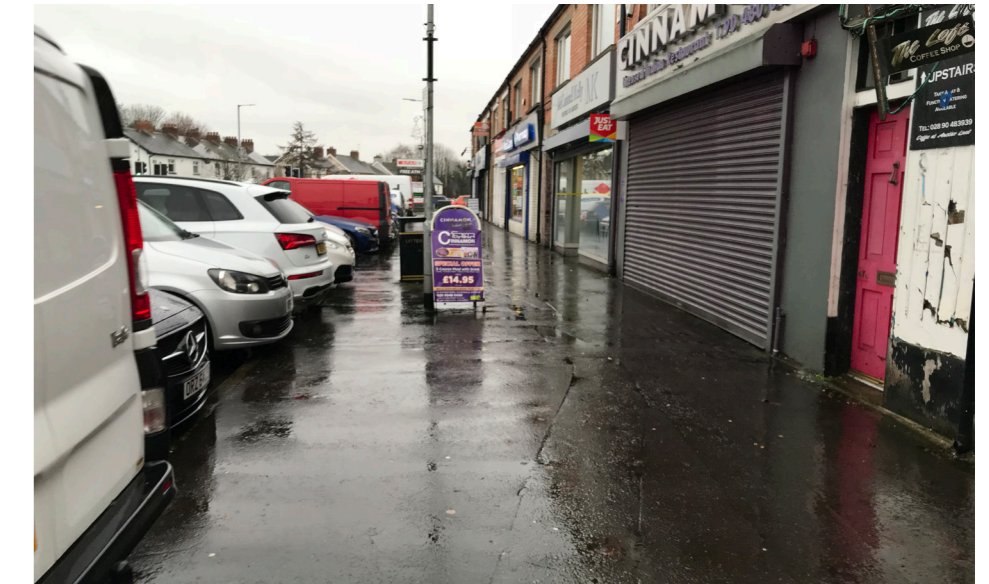
View of existing paving along Comber Road
