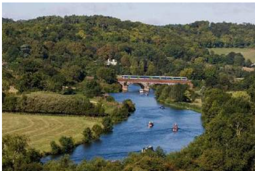
Figure 11 Brunel's rail viaduct at Gatehampton
