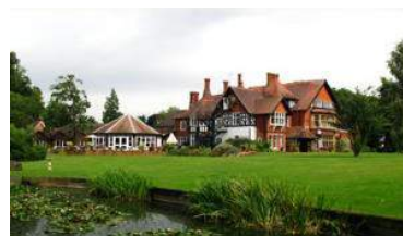
Figure 66 The Grange, nineteenth century, now care home
