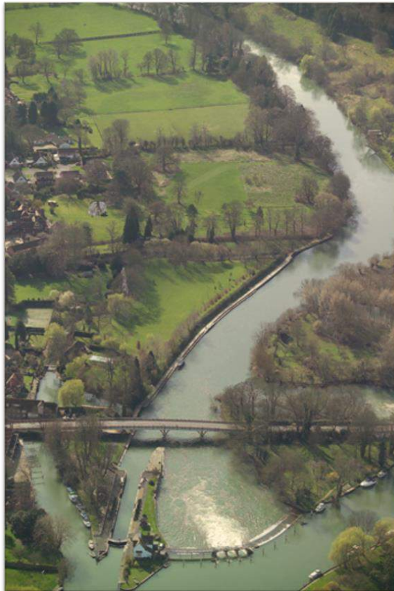
Figure 51 Goring weir and southwest floodplain
