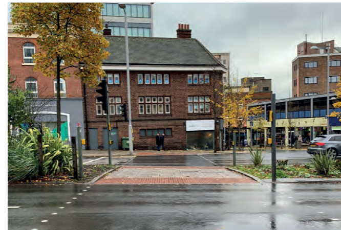
Maid Marian Way, Nottingham Supercrossing – direct, wide crossing and integrated green features (Photo credit: MottMacdonald)
