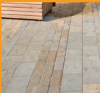
A combination of high quality concrete and stone paving to footpaths (Scoutmoor setts/conservation x)
