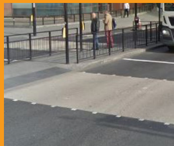
Coloured Asphalt on Cycleways / Pedestrian Crossing Points (Light Buff UltiColour Asphalt)
