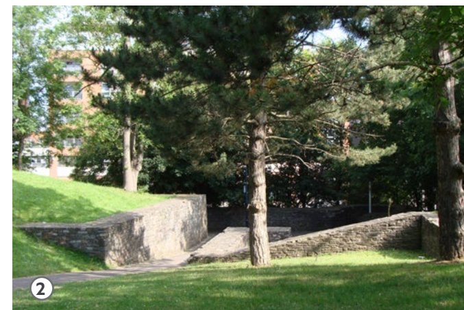
Fig. 89 Existing walls within Castle Park
