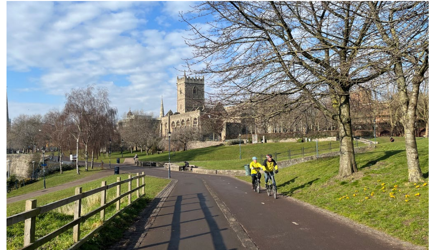
Fig. 114 Site Photo - Existing cycle path to Floating Harbour. The adjacent footpath is narrow and there is a lack of delineation between the routes.
