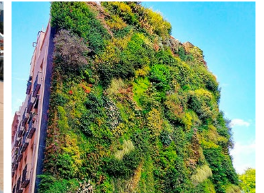
Frontage to Castle Park - Biodiverse Vertical Greening
