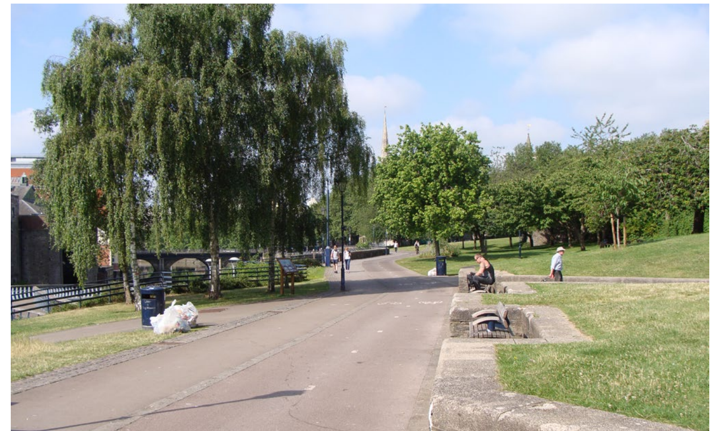
Fig. 115 Site Photo - Existing cycle path to Floating Harbour with benches facing onto the cycle path. The adjacent footpath is narrow and there is a lack of delineation between the routes.
