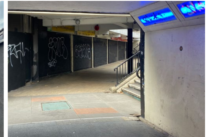
Subway ends in area with limited inter-visibility
