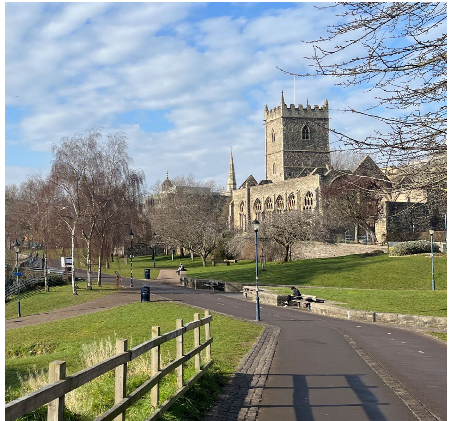
Fig. 12 Site photo looking towards St Peter's Church from Castle Park
